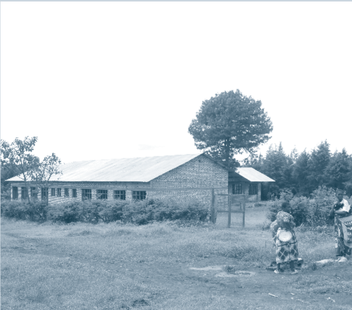
Work on the new school buildings progresses
